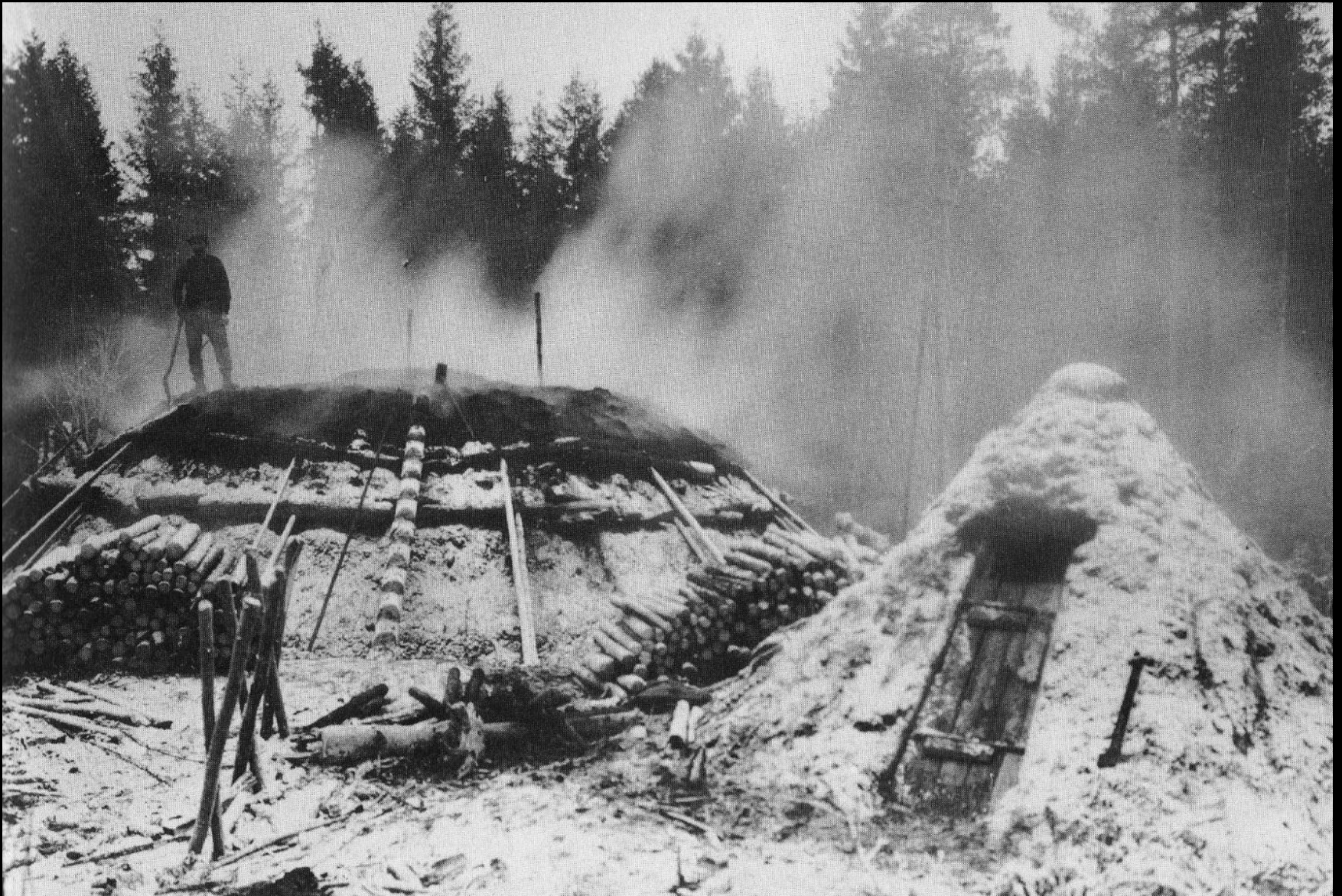
One charcoal stack was needed for every 24 hours of operation at the blast furnace
