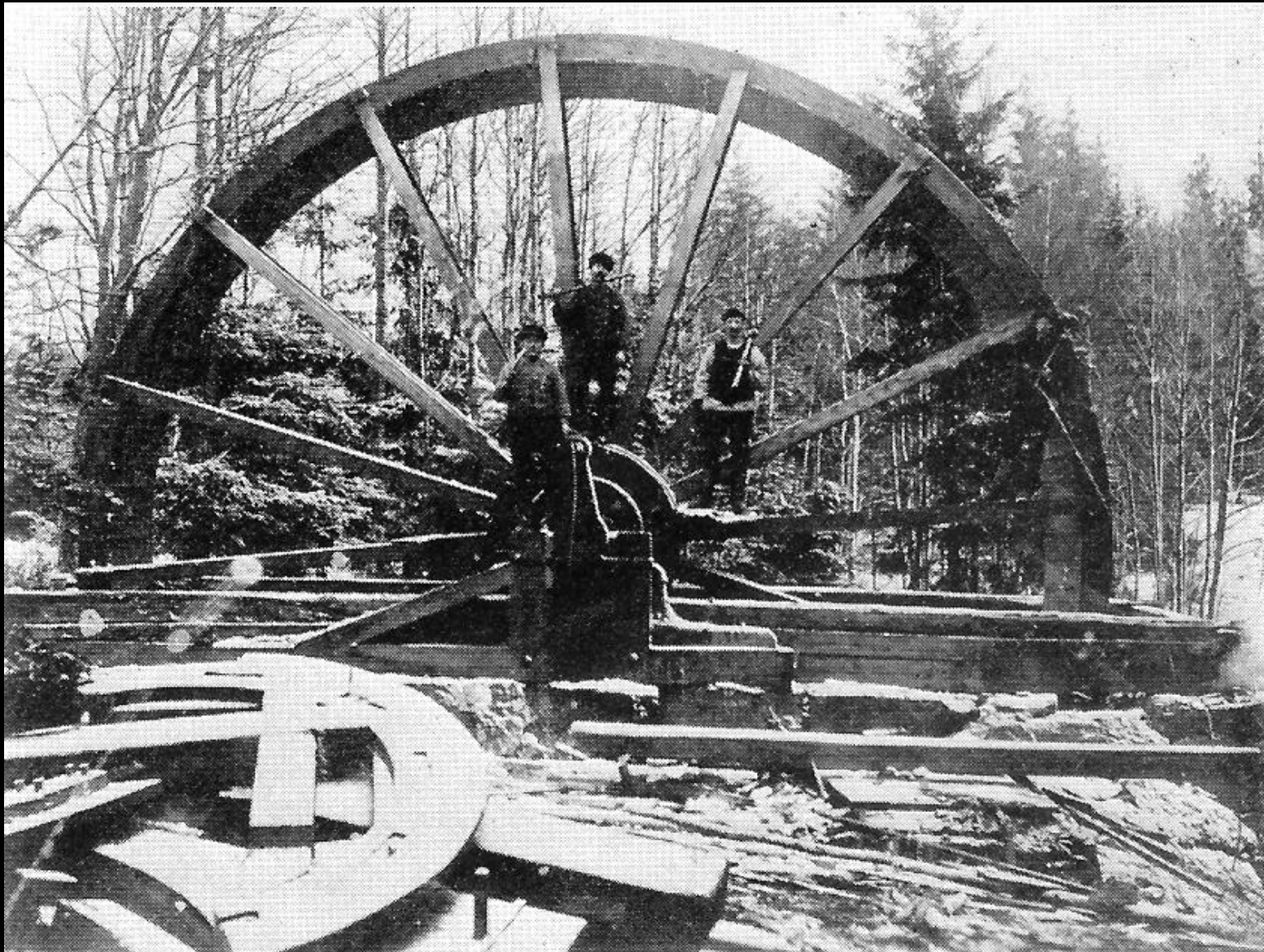
One so called "water art" to move water power to the mine
