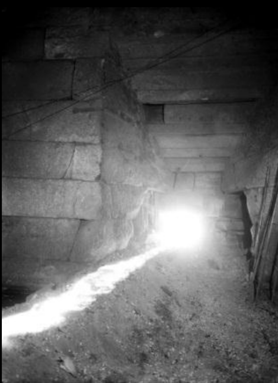
The outflow of iron and slag at what was called the "breast"
